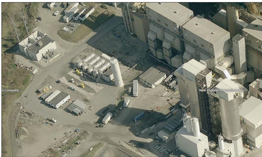
4 x 55,000 Gallons Aqueous Ammonia SS 304 Storage tanks
